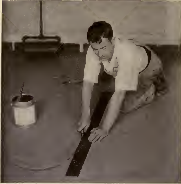
CUTTING JOINTS AND MATCHING SEAMS
